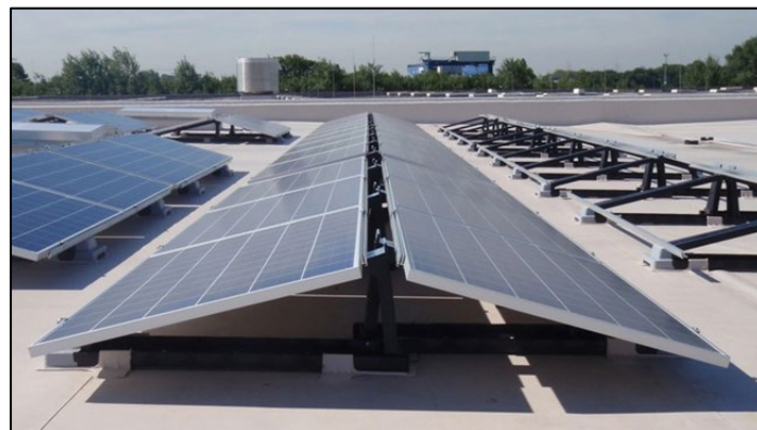
Figure 3: Rooftop Solar Photovoltaic (PV) Design
