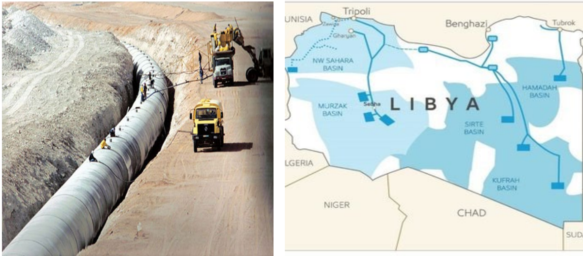
Figure 5. Artificial river in Libya to bring water from desert aquifers to the coast [6].
