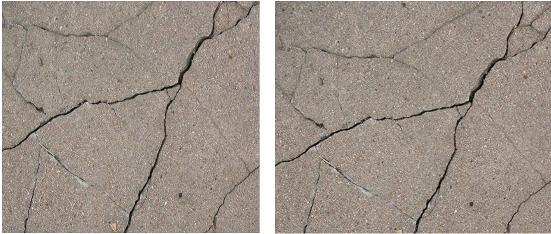
Figure 4. Non-Structural Cracks [5].
